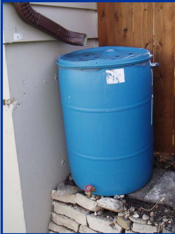
A simple rain barrel with intake from a downspout (top), a drainage spout (bottom), and an overflow spout (side). Note that a hose should be attached to the overflow spout to drain water away from the house foundation.
